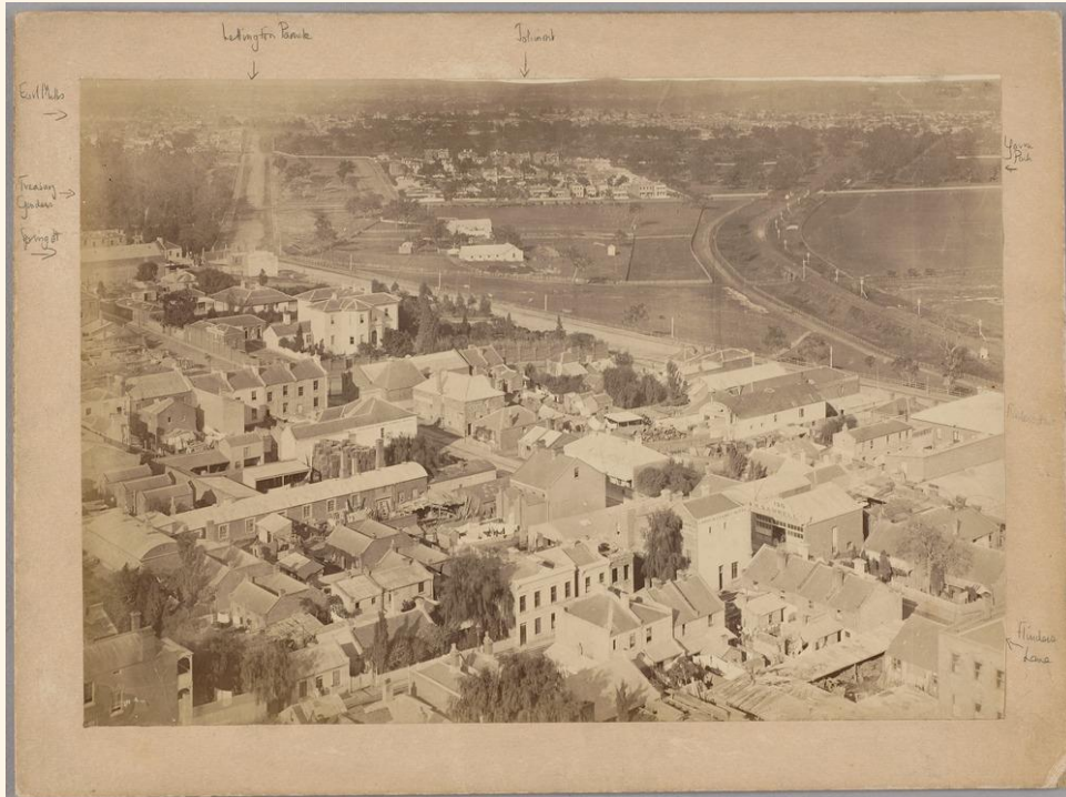
'[Looking south-east from the spire of Scots Church, showing Flinders St., Wellington Parade and Jolimont]'. George Porter's Cleveland House is on the far side of the large two-storied white house with a garden fronting Flinders St., near the corner of Exhibition St. (top left). Paterson Bros Photographers, 1875. State Library of Victoria H8007 file b47464
